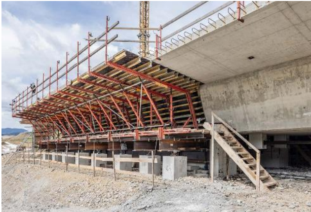
The VIL Incremental Launching Facility impressed with its high load-bearing capacity, leading to time and material savings.
