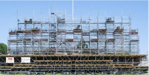
The 26-m high rear tower was a complex structure as it could not be braced and anchored in the usual way. There was also a historical statue in the middle of the scaffolding that needed to be protected.
