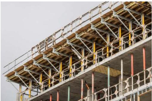
Image above: The combination of SKYTABE and BR Shaft Platforms ensured an accelerated process, as the systems could already be installed on the next storey.
