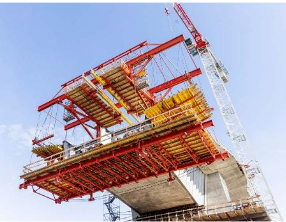
The balanced cantilever carriage was delivered pre-assembled and just-in-time, which freed up valuable space on the construction site.
