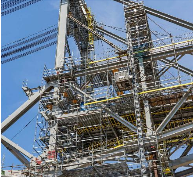
The flexible 25-cm grid size of the PERI UP Modular Scaffolding also enables complex scaffolding.
