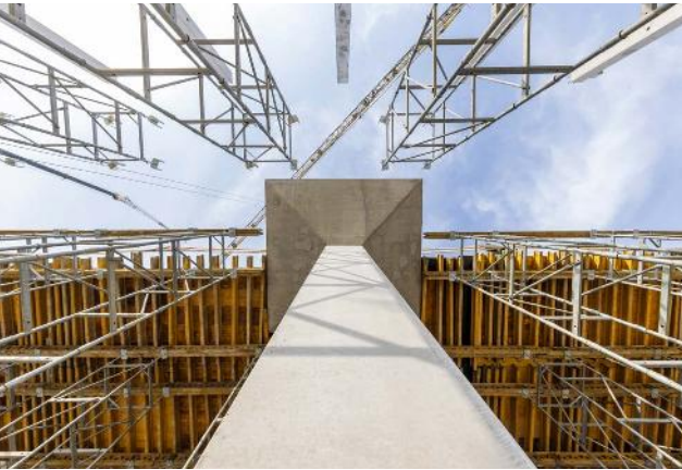
A combination of several formwork systems provided the central building block for the prefabricated columns with bases in the second and third sections of the hall.
