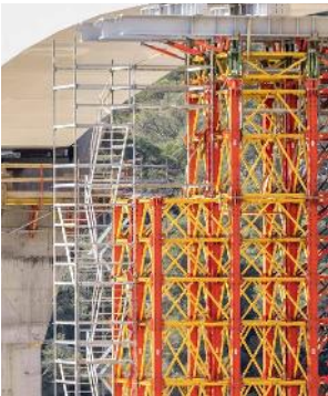
The PERI UP Stair Tower provided a safe and convenient means of access to the top.
