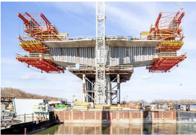
By using the VBC Formwork Carriages, it was possible to build the bridge efficiently using the cantilever construction method with a shorter construction time.
