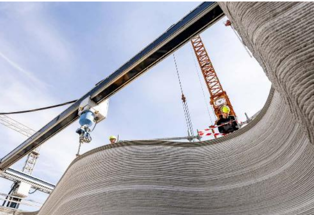
Using the COBOD BOD2 3D Printer, the wave-shaped facade of the 9-metre high building was printed in just 170 hours.
