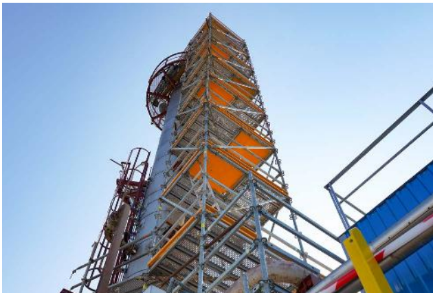
The 18-m high stair tower was firmly anchored to the steel structure and provided a safe and stable route to the MTBE column.
