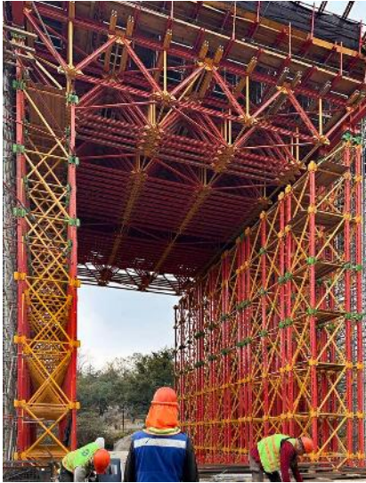
Due to the low weight of the ALPHAKIT Steel Components, the parts could be completely assembled by hand - without any lifting equipment.
