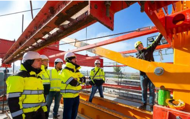
To ensure a smooth construction process, the customer received technical support from PERI Experts on the construction site near Nowy Targ.
