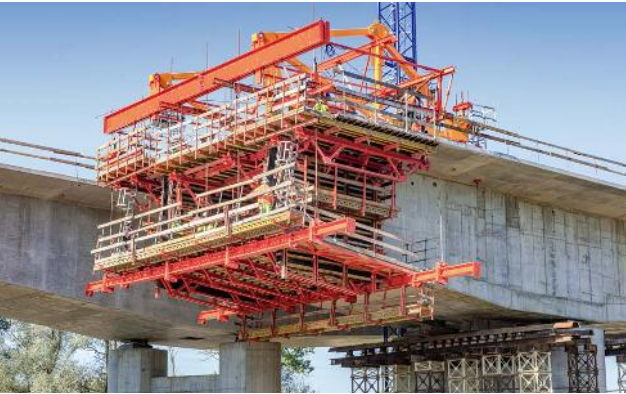
To meet the weekly concreting cycle, segments of up to 5 m in length per section were formed using the VBC Balanced Cantilever Carriage.
