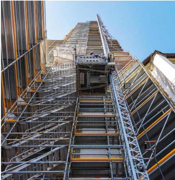
Above the heavy-duty platform, the scaffolding elevator and stairs enabled access all the way up to the onion-shaped tower top.
