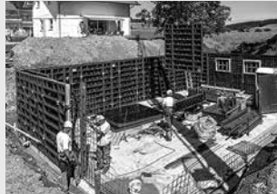
Wall Formwork
