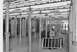
Slab Formwork
