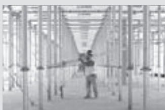
Slab Formwork
